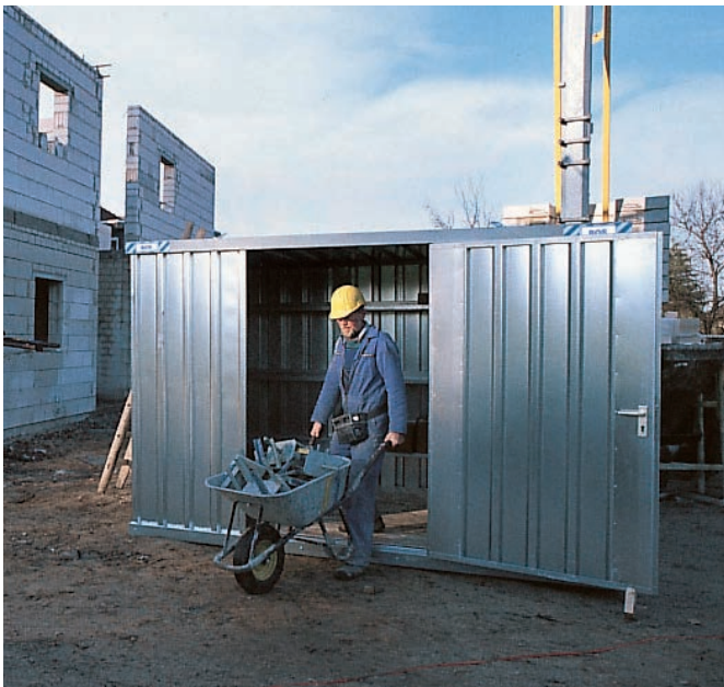
Building site container
