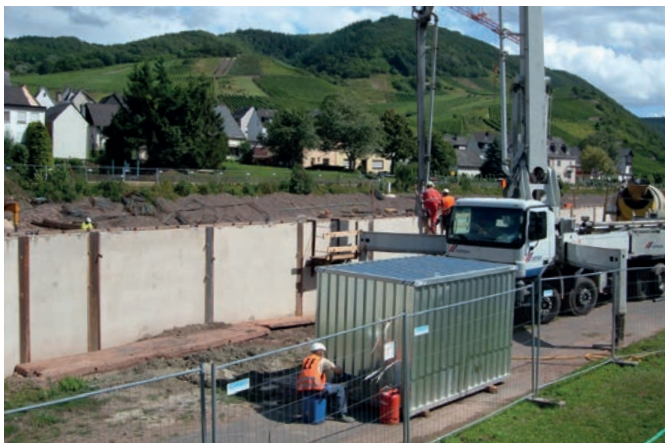
SC3000 on a construction site
